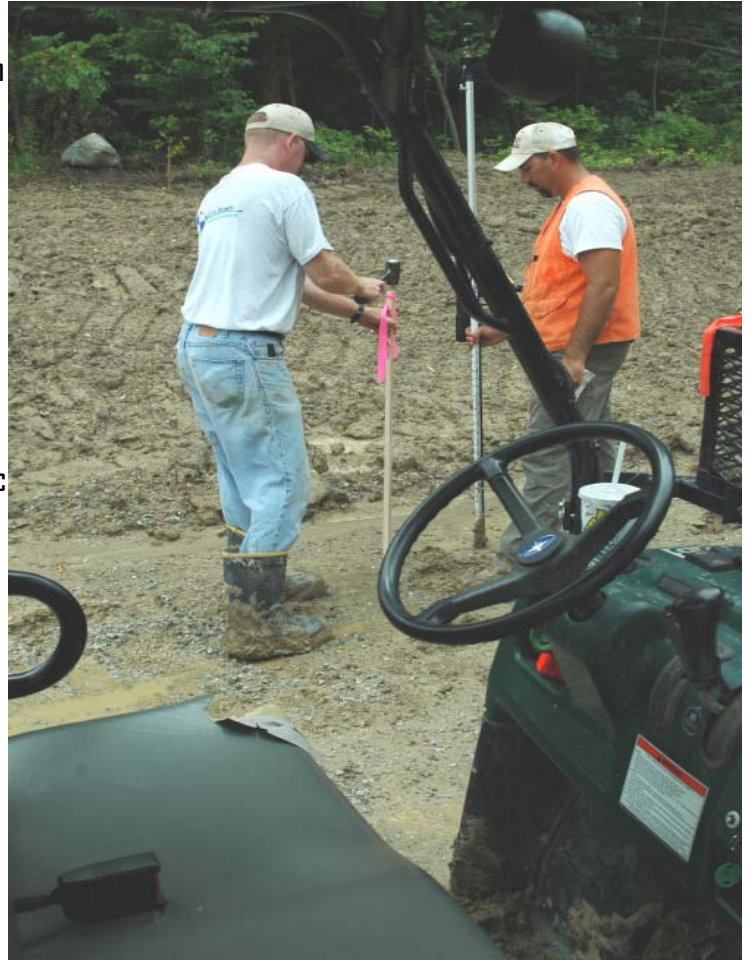
Field crew staking with robotic station and Ranger ATV
