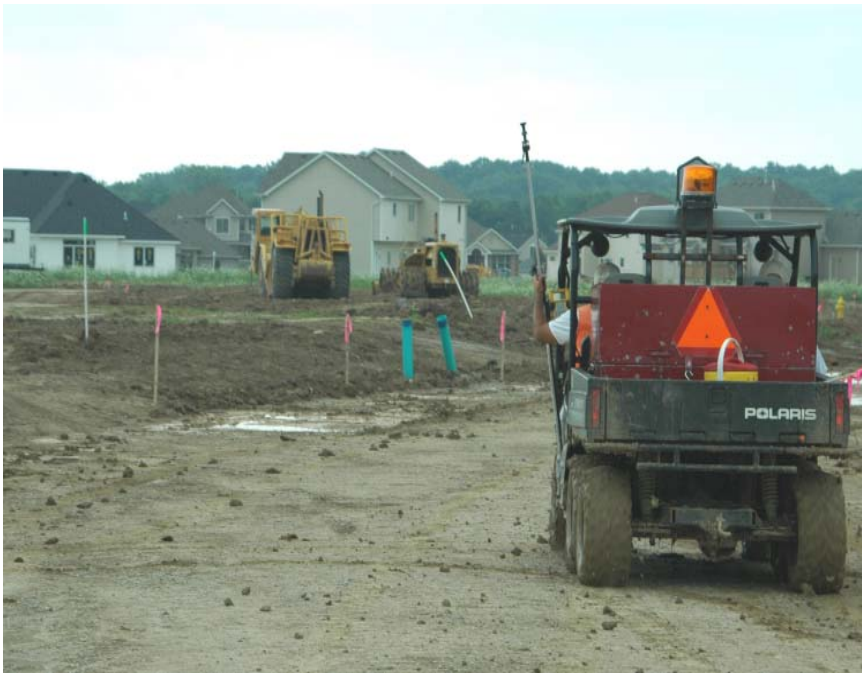
Typical construction staking site with Ranger ATV
