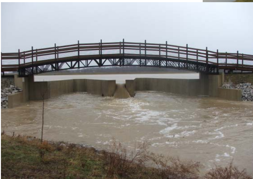
Dam, Weir, and Footbridge during heavy flooding event
